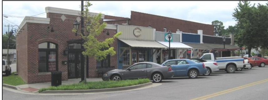
Several commercial brick buildings appear to have been encased with EIFS (exterior insulation finishing system).
